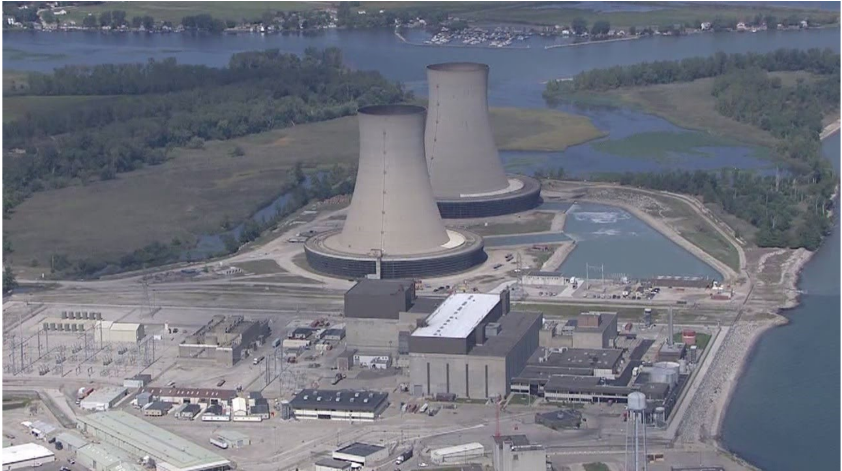
DTE Energy – Enrico Fermi Nuclear Plant – Newport, Michigan
