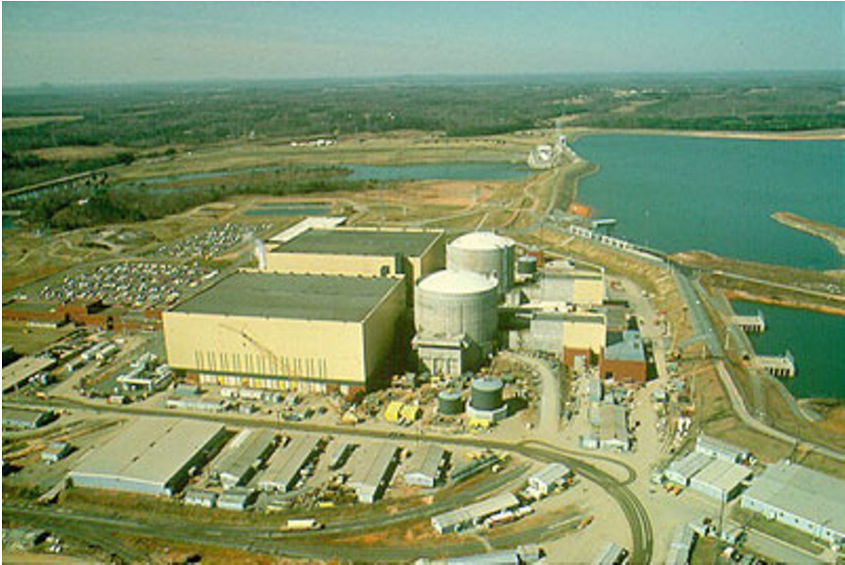
Duke Energy – McGuire Nuclear Station – Huntersville, North Carolina
