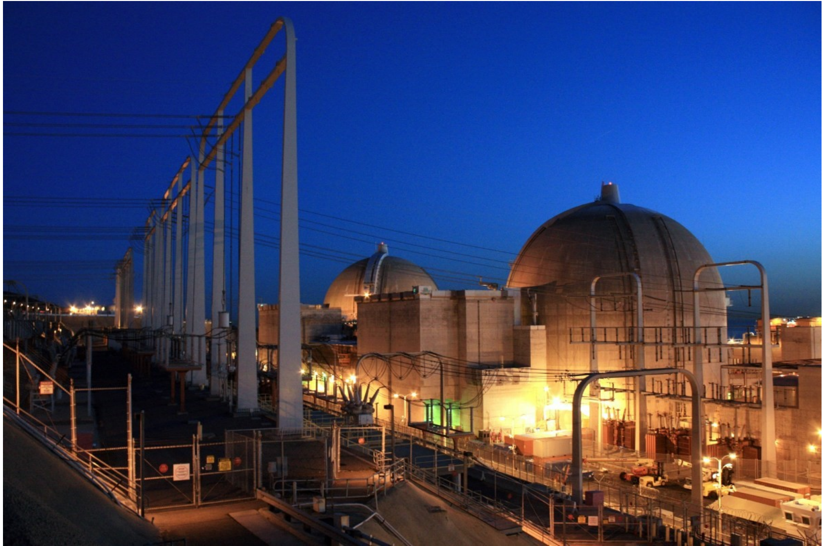
San Onofre Nuclear Generating Station Units 2 and 3
