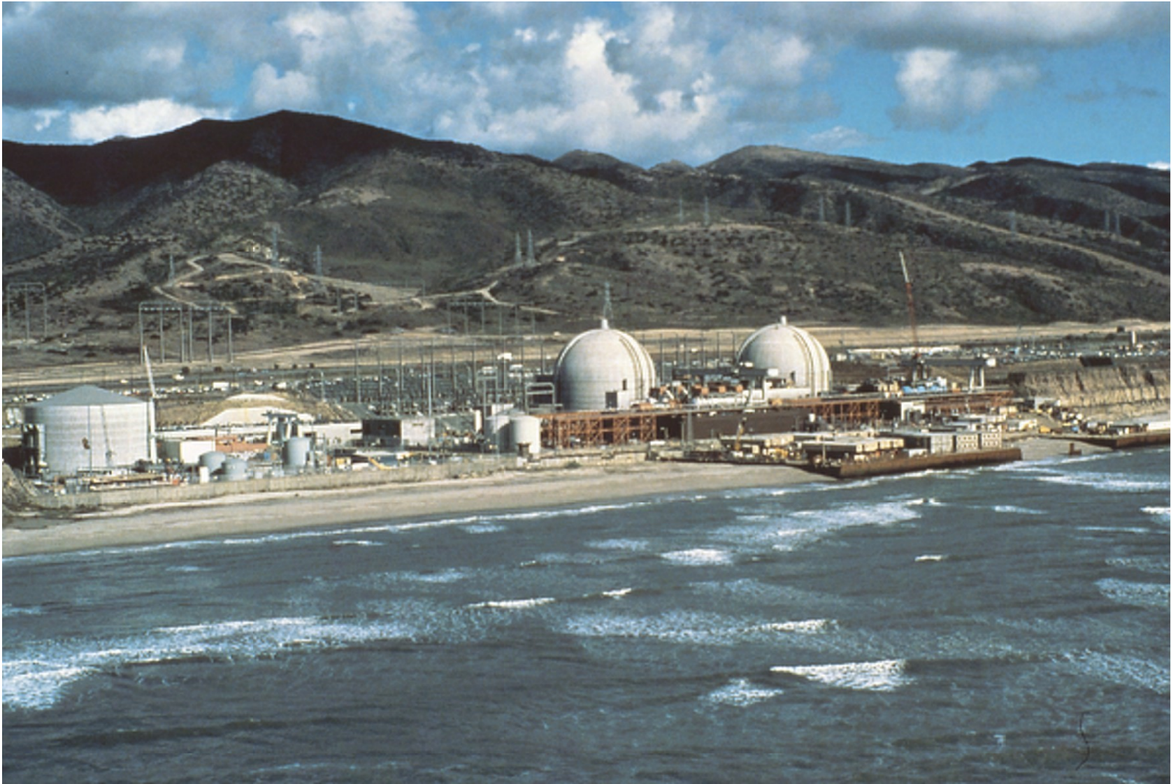
San Onofre Nuclear Generating Station Units 1, 2, and 3
