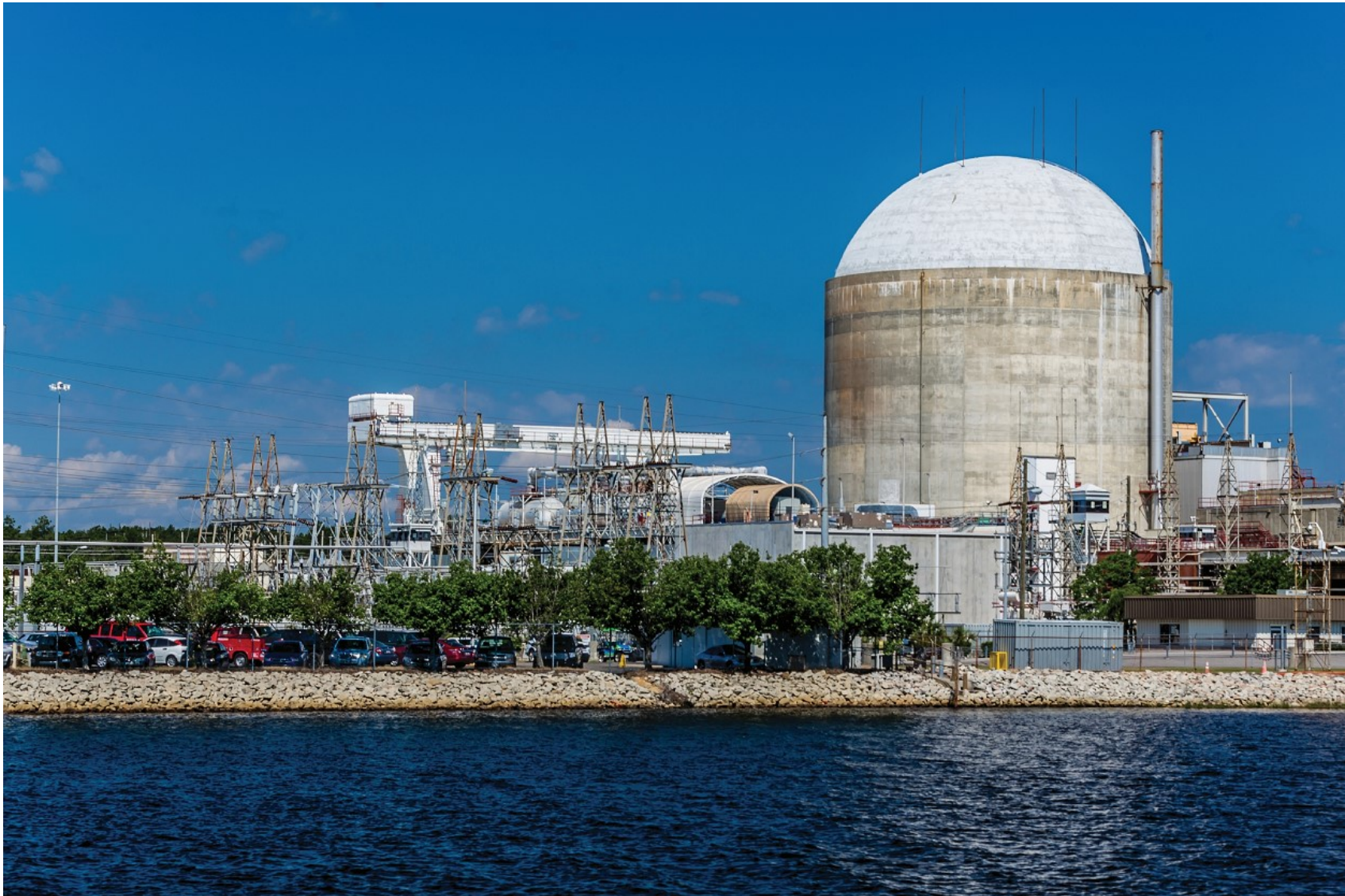
Duke Energy – H. B. Robinson Nuclear Plant – Hartsville, South Carolina
