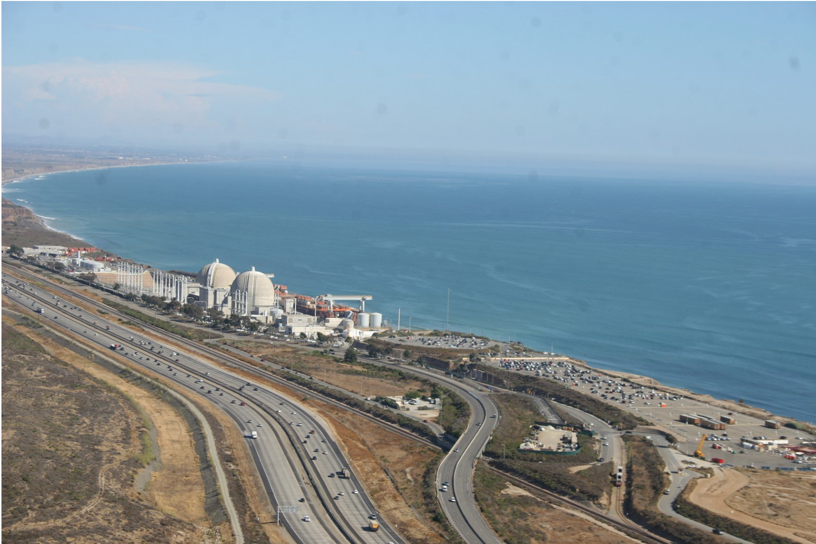
San Onofre Nuclear Generating Station – San Clemente, California
