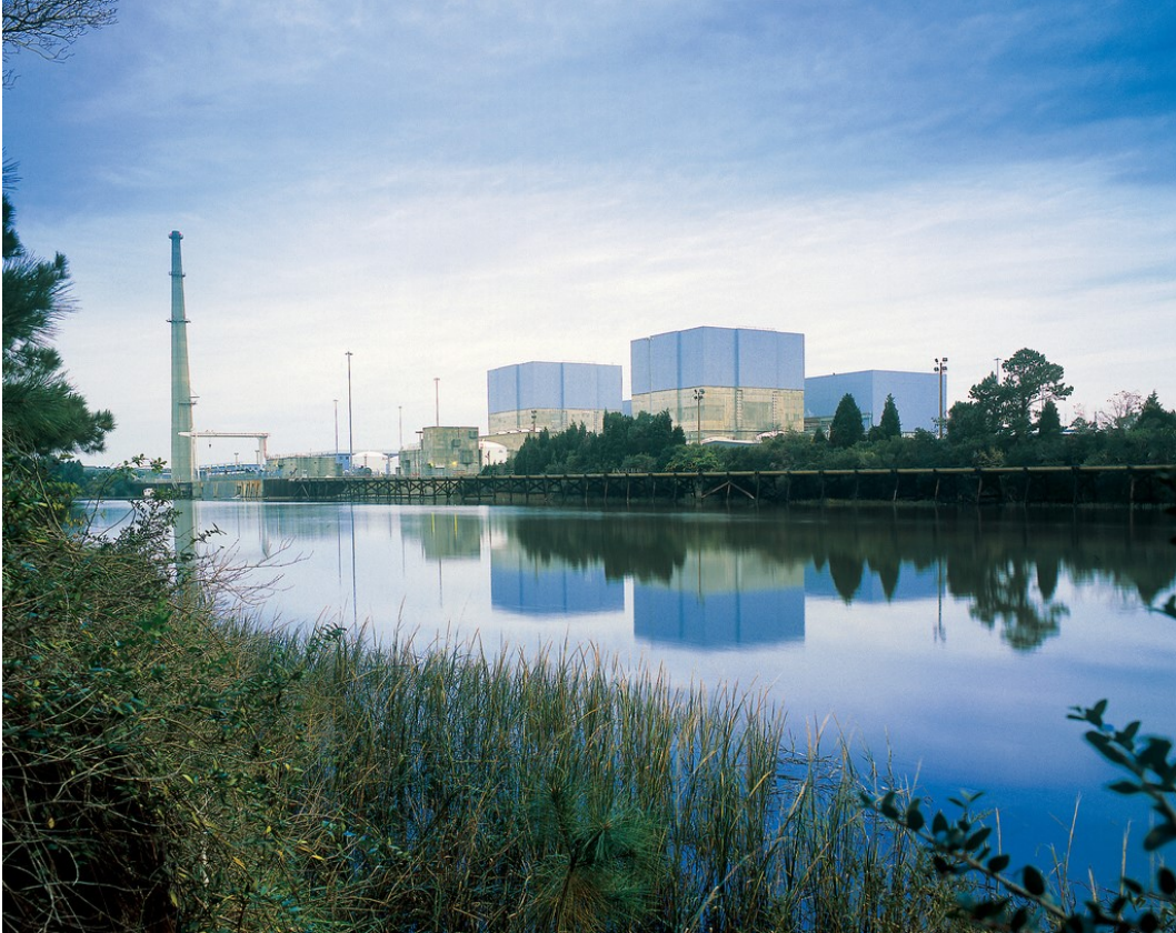
Brunswick Nuclear Plant – Southport, North Carolina
