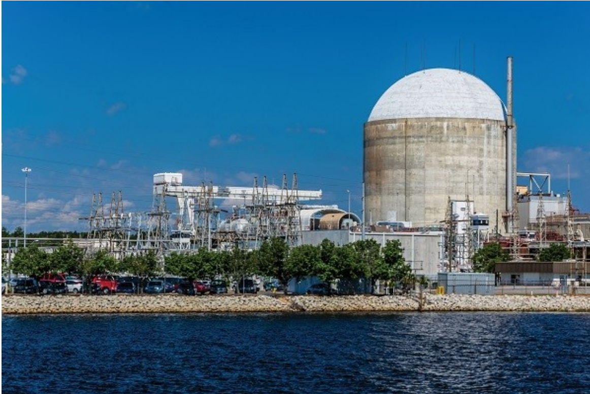
H. B. Robinson Nuclear Plant – Hartsville, South Carolina
