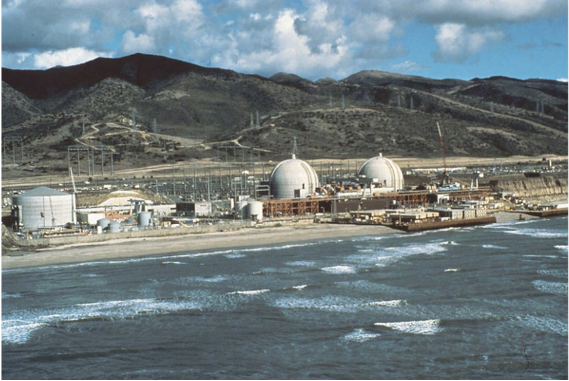
San Onofre Nuclear Generating Station Units 1, 2, and 3
