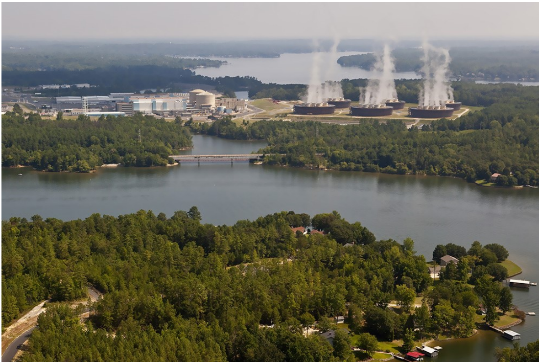
Catawba Nuclear Station – York, South Carolina
