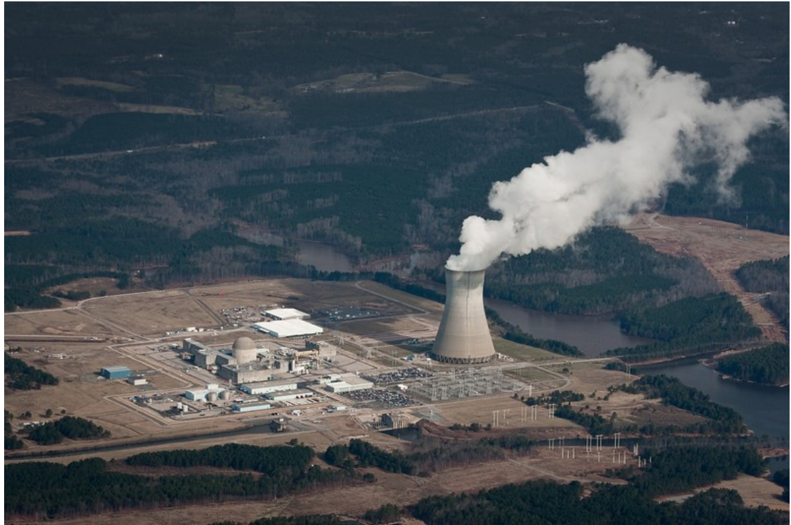
Shearon-Harris Nuclear Plant – New Hill, North Carolina
