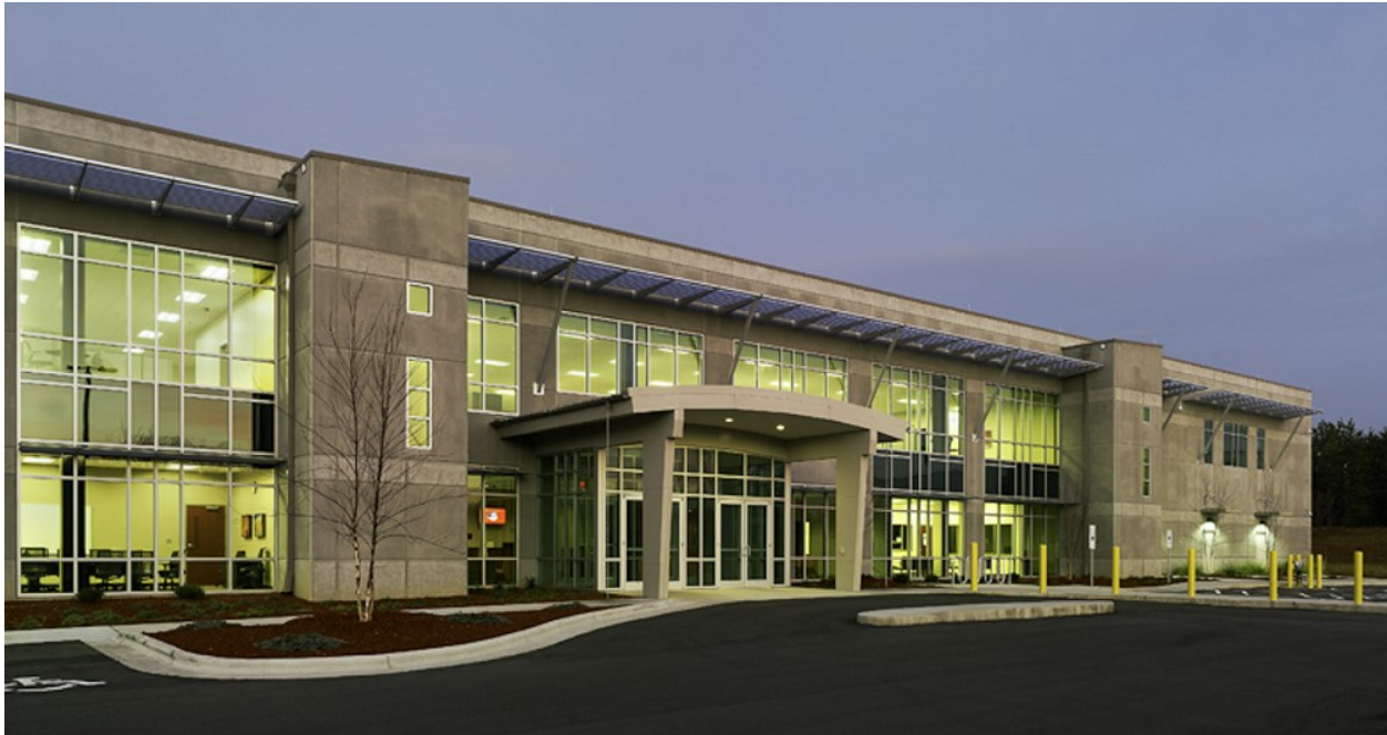
Duke Energy Generation Support Facility Kings Mountain. North Carolina
