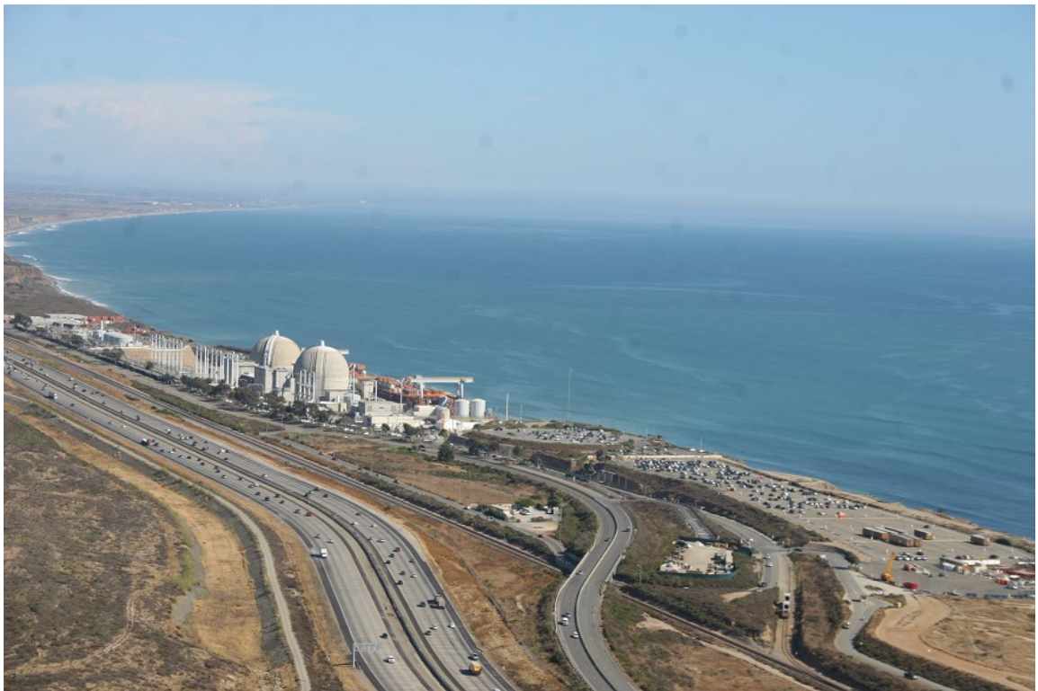
San Onofre Nuclear Generating Station Units 2 and 3 and Pacific Ocean
