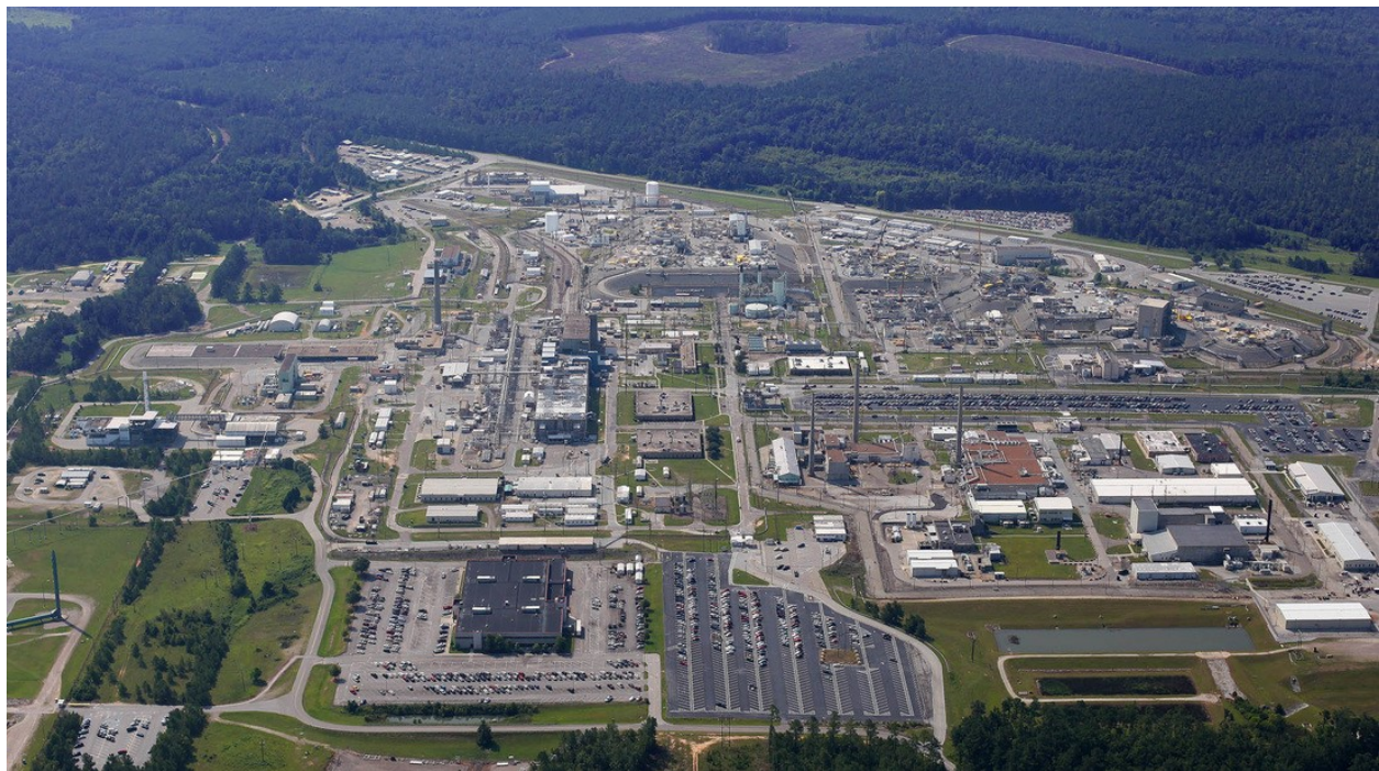
Savannah River Site – H Area United States Department of Energy Savannah River Site Aiken, South Carolina
